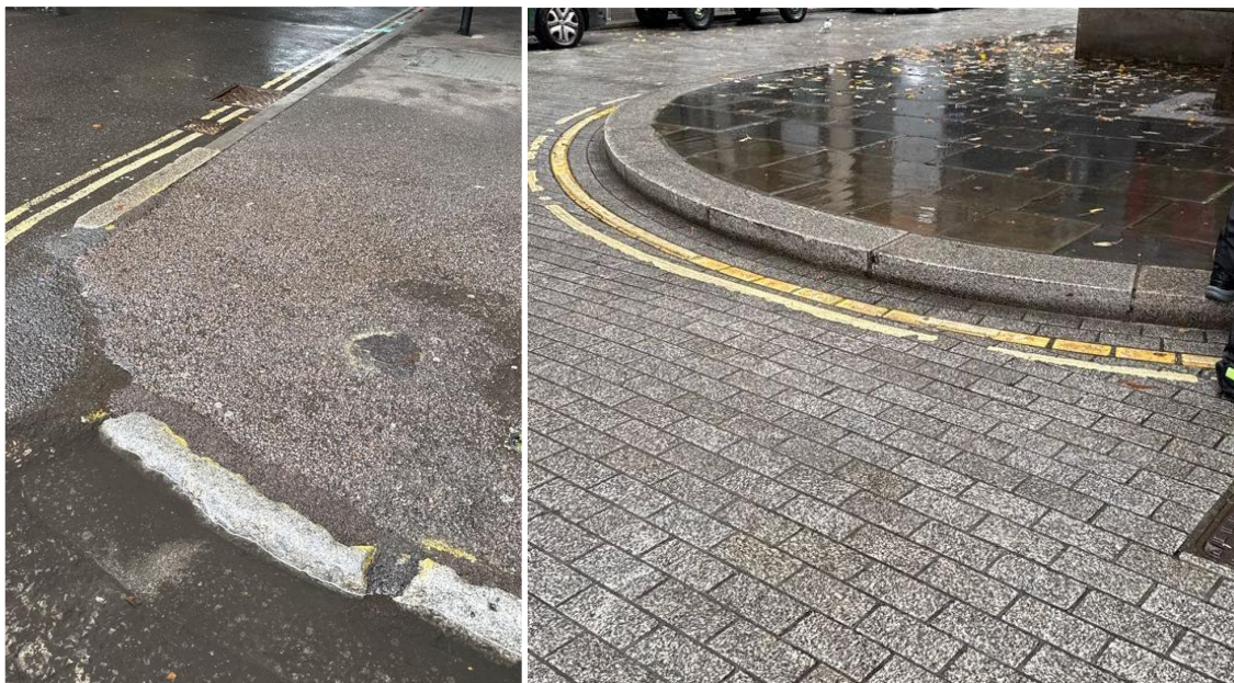
Image 1: Dropped kerb that hasn't been maintained.
